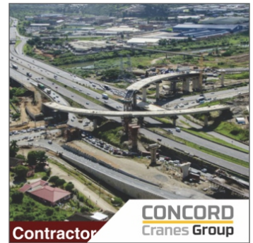
Contractor CONCORD Cranes Group NEW ROAD INTERCHANGE Date Completed: 1996
