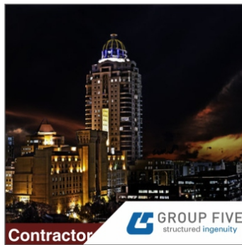
Contractor GROUP FIVE structured ingenuity MICHELANGELO TOWERS Date Completed: 2003
