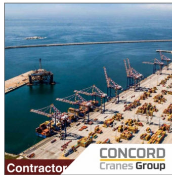
Contractor CONCORD Cranes Group KOEGER HARBOUR Date Completed: 2004
