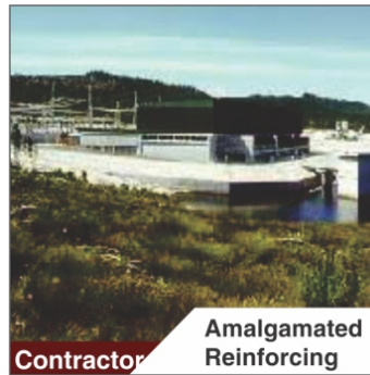
Contractor Amalgamated Reinforcing GRABOUW PUMP STATION Date Completed: 1987
