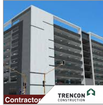
ELLIS PARK PARKADE Date Completed: 2009
