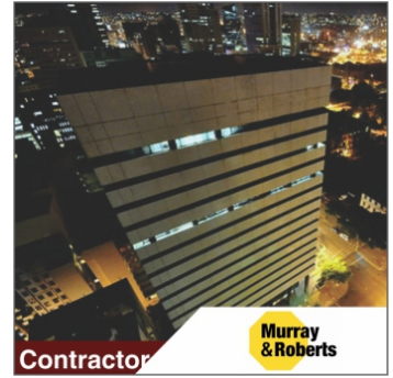
Contractor Murray & Roberts SHELL HOUSE Date Completed: 1974
