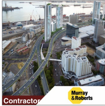
Contractor Murray & Roberts FORESHORE FREEWAY PROJECT Date Completed: 1974
