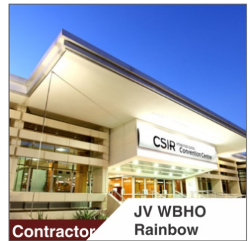
Contractor JV WBHO Rainbow CSIR PRETORIA Date Completed: 2004
