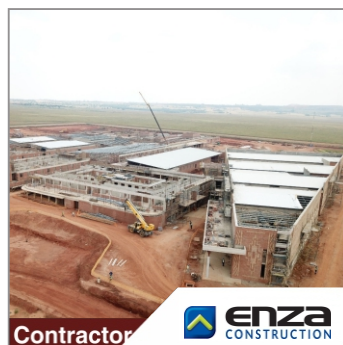
MIDDLEBURG HOSPITAL Date Completed: 2020
