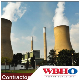
Contractor WBHO RELY ON OUR ABILITY SASOL COOLING TOWERS Date Completed: 2004
